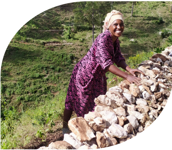
A Haitian farmer constructs a mechanical barrier to protect the hillside from erosion.
